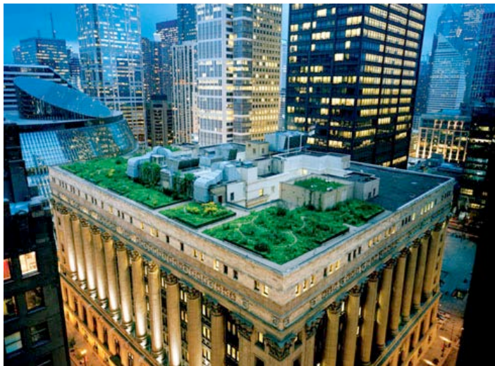
FIGURE 3-4 – Chicago City Hall Green Roof
