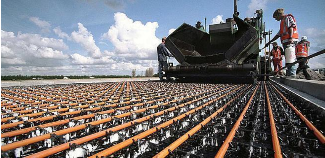
Figure 7-5 Geothermal de-icing
